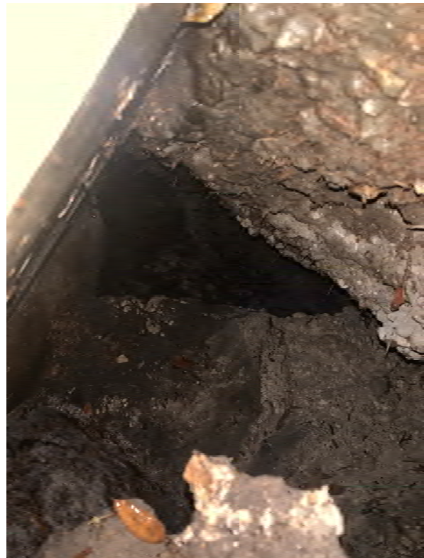
Photo 3. Looking inside small opening at void around pipe connection at inlet 11-48.
